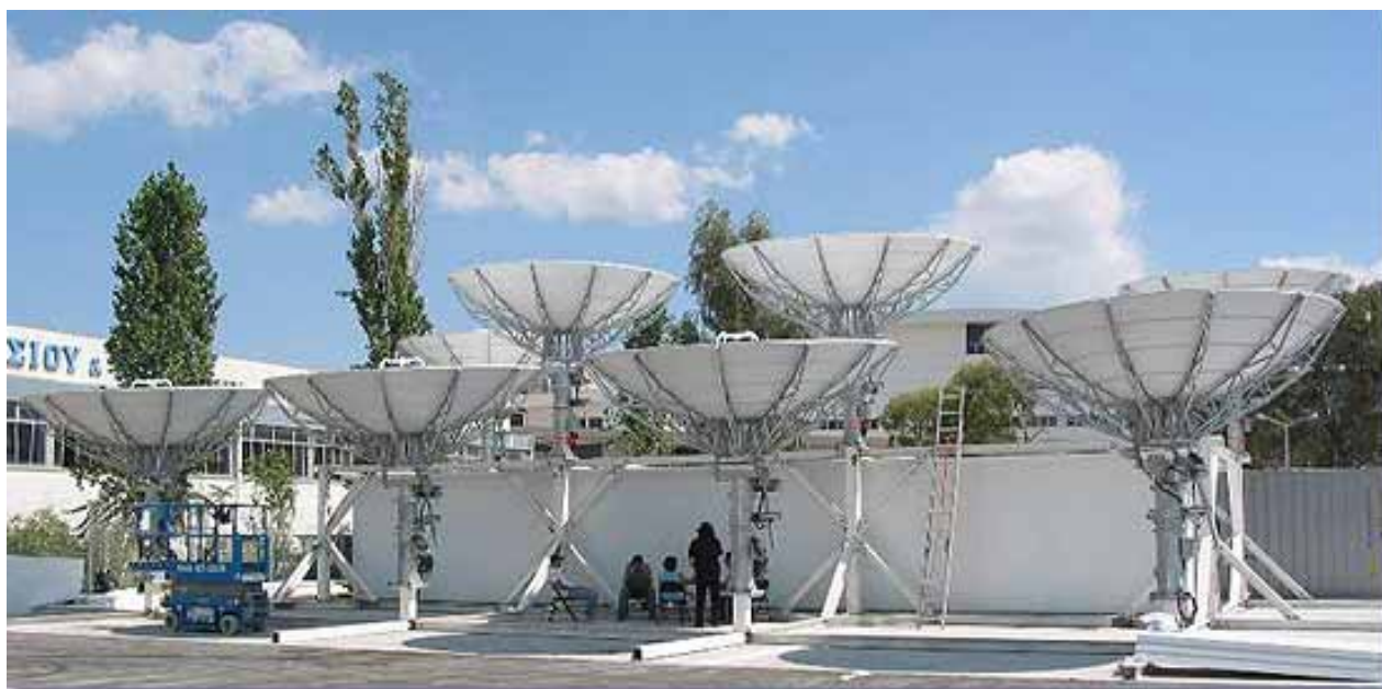
Satellite dishes on site
